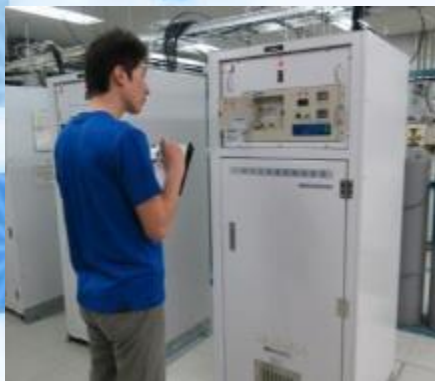
Operation of GAW Station
